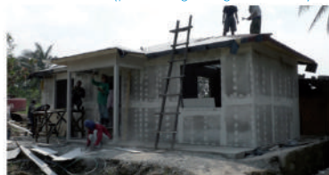
PUTTY APPLICATION (joints and screws)
