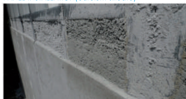
PARTITION WALLS (panels + lightweight concrete)
